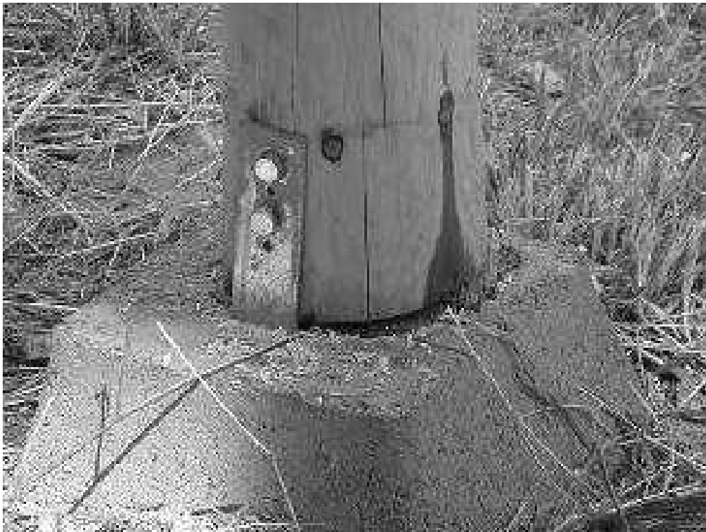
Figure 7 Post to pier pad attachment details
