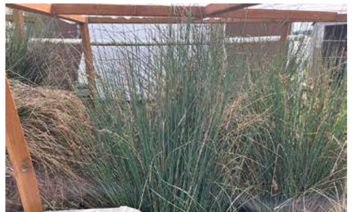
The greywater filtration system at Community Supported Shelters' Skinner Community.
