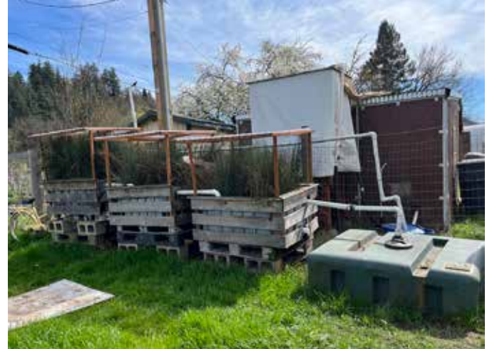
Native aquatic plants help filter the water in the greywater systems at CSS community sites.
